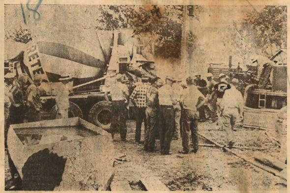
Pictured above is the machine which was used to cement the casing of the new Strart well. Two of the ready-mix trucks used to haul the bulk cement can also be seen in the picture. Before work could be started all trucks had to be at the well site because when once they start they cannot stop until the job is completed.
