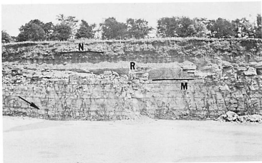
Figure 8. Nora(N), Rock Grove(R), and Mason City(M) Members in the Williams quarry; arrow marks position of discontinuity surface shown in figure 9.
