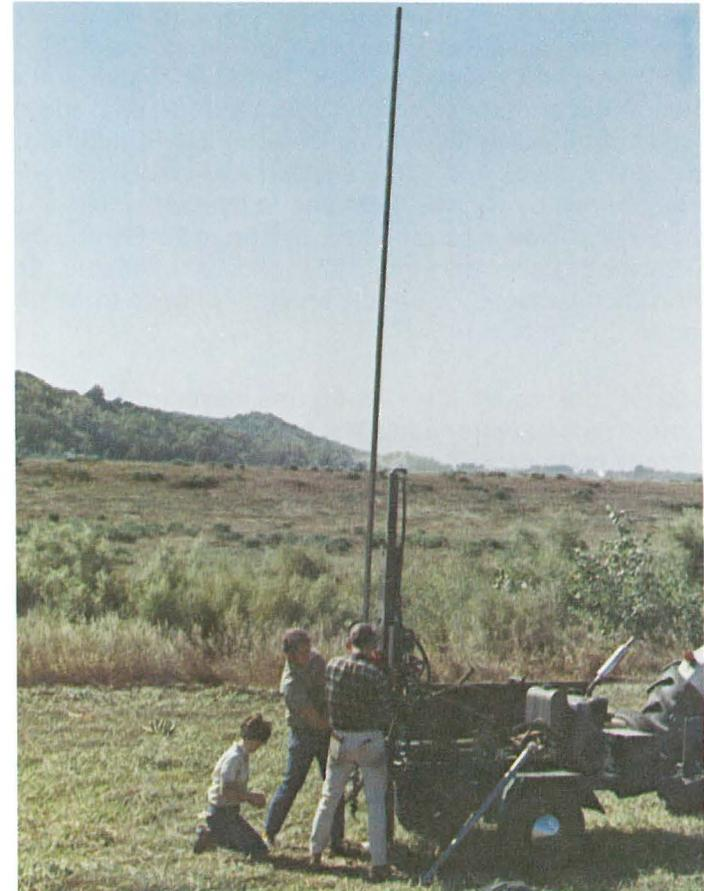
Figure 9. Drilling projects provide information on types of sediments that lie beneath the land surface. Here, along Waubonsie Creek in Fremont County, samples are taken to determine whether the sediments were deposited by the Missouri River, out of the picture to the right, or whether they originated from the loess hills in the background. Photo by James C. Davis.
