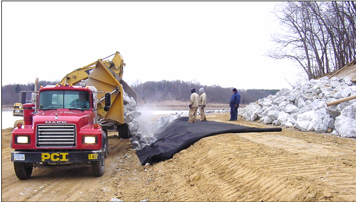
Figure 22. Side-dump semi-trailer dumping armoring stone on landscaping fabric. The end loader behind the truck moved the rock into place. Photo by Paul Sleeper.
