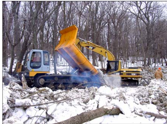
Figure 23. Smaller, tracked rear-dump trucks were employed to transport stone to less accessible areas of the Lake Macbride shoreline. Photos by Paul Sleeper.
