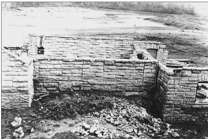
Figure 17. The partially dismantled old bathhouse. The structure was disassembled stone by stone and reconstructed above the new beach.
