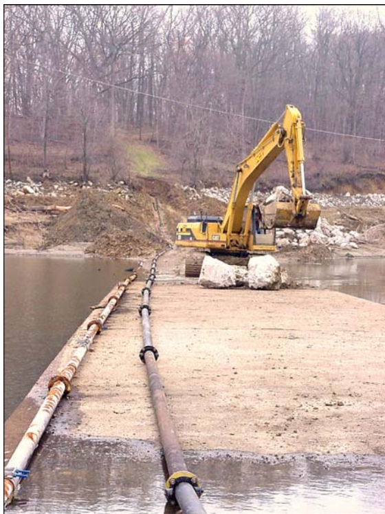
Figure 24. Old and new pipeline carrying treated sewage from the Cottage Reserve area
