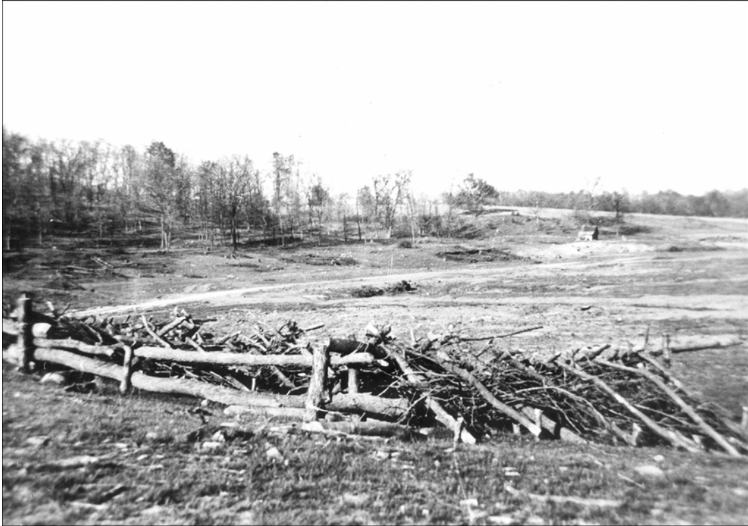
Figure 7. CCC workers constructed fish habitat prior to filling Lake Macbride in 1934.
