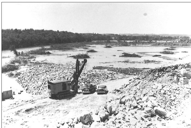
Figure 15. Construction work raising the level of the Lake Macbride dam in the mid- 1950s. Flooding of the new Coralville Reservoir had already begun and can be seen in the background.
