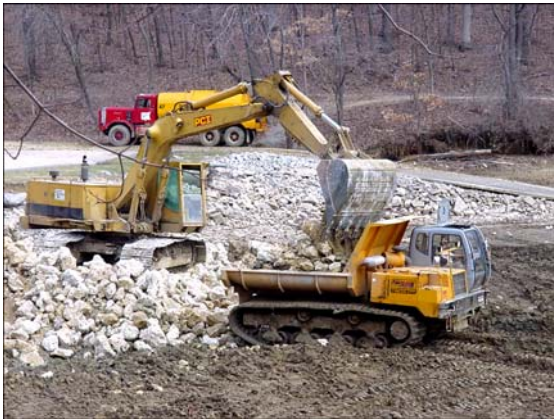
Figure 23. Smaller, tracked rear-dump trucks were employed to transport stone to less accessible areas of the Lake Macbride shoreline. Photos by Paul Sleeper.
