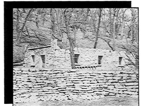
Hatchery building, completed in 1939, of natural rock laid edgewise in concrete to blend with rock surroundings of Big Spring.
