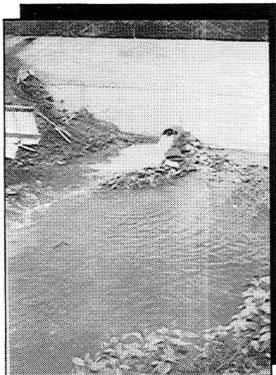
18-by-94 foot section of dam base with 30-inch tube for water flow during dam construction in 1938.
