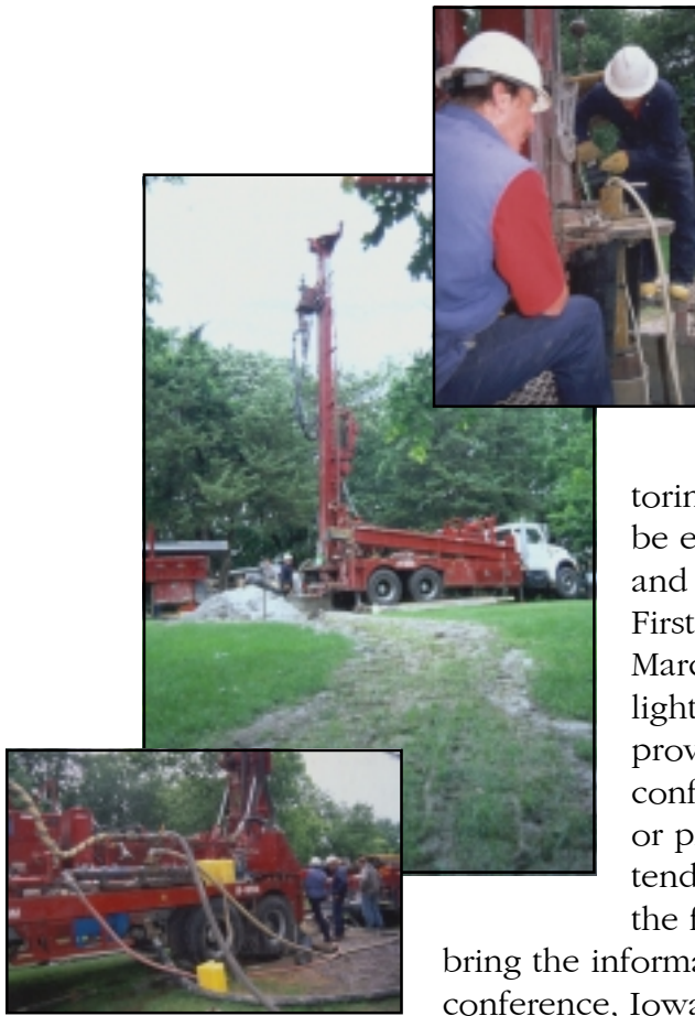
Figure 5. Drilling a groundwater well at Briggs Woods County Park, Hamilton County.
