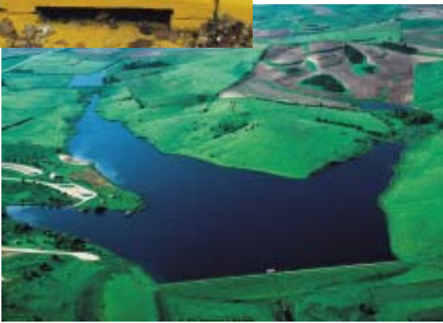
A watershed dam and upland terraces in a small watershed project in western Iowa.
