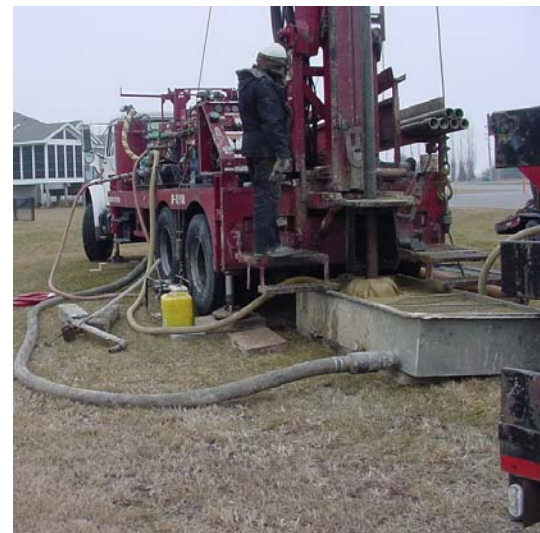
Drilling of bedrock wells at Westfield Elementary School, Linn County.
