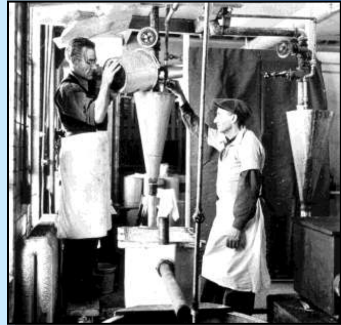
Army Kitchen Waste Systems
